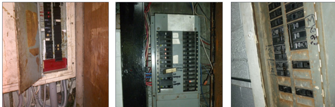
Figure 10 Older electrical panels, such as these examples, may require upgrades to meet today's electrical codes
