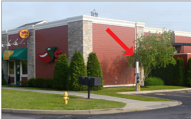
Figure 6. These charging station installations (noted by red arrows) are sited in convenient, but not prime parking spaces that minimize conduit runs to reduce costs Courtesy Energetics Incorporated
