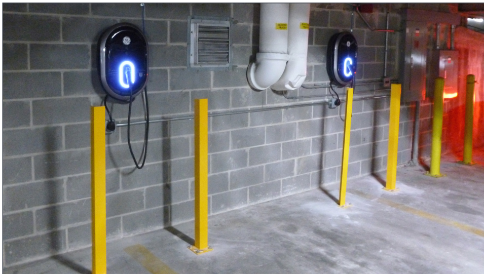
Figure 16. Bollards, tire stops, and sign posts can be used to protect charging stations and electrical cords from physical damage
