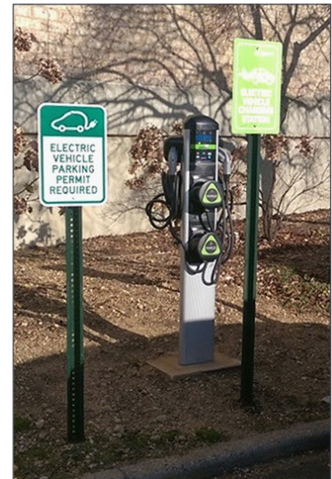
Figure 16. Bollards, tire stops, and sign posts can be used to protect charging stations and electrical cords from physical damage
