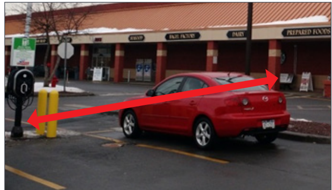
Figure 7. Charging stations at parking spaces away from a building require longer trenching through pavement (red lines indicate distance) and could disrupt traffic flow during construction! Courtesy Energetics Incorporated
