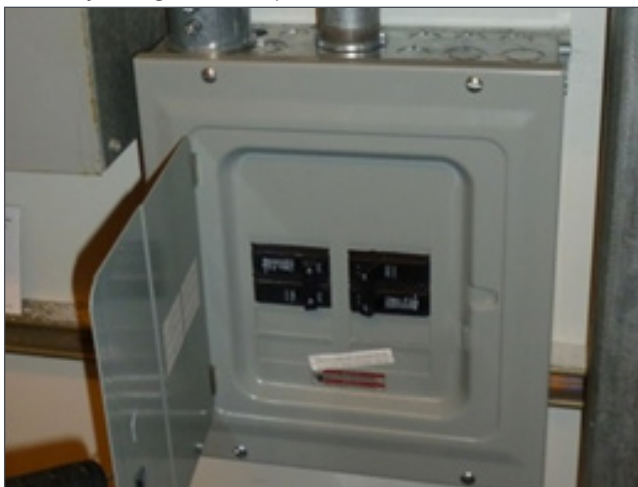
Figure 12. Charging station circuits may require an added subpanel, such as this one, if space in the main panel is limited
