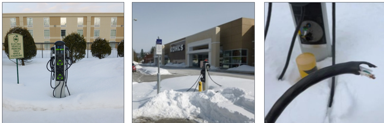
Figure 9. Snow management practices must be considered because snow accumulation can obstruct access to EV charging and snow plows can cause damage to charging stations
