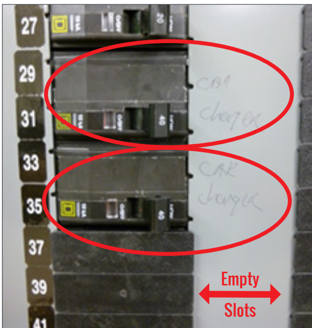
Figure 12. Charging station circuits may require an added subpanel, such as this one, if space in the main panel is limited
